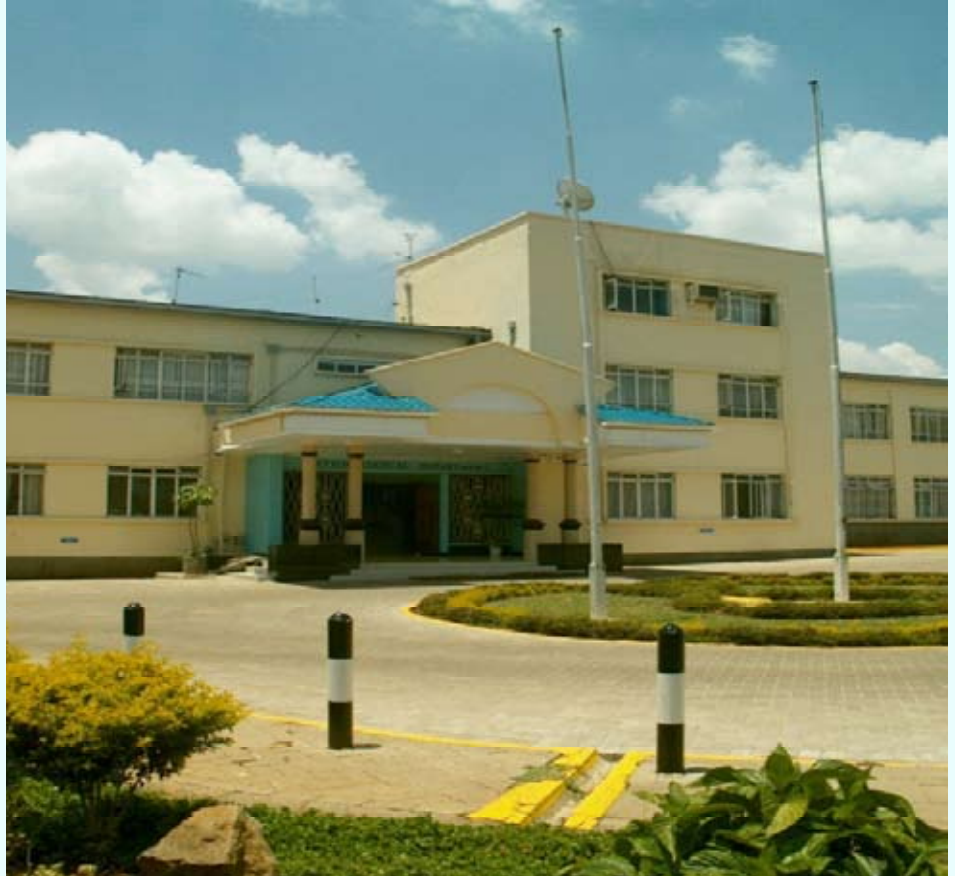
The Kenya Meteorological Department headquarters.
